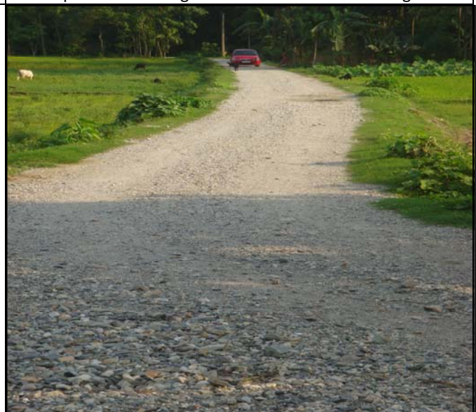
Condition of the road near the PWD road
