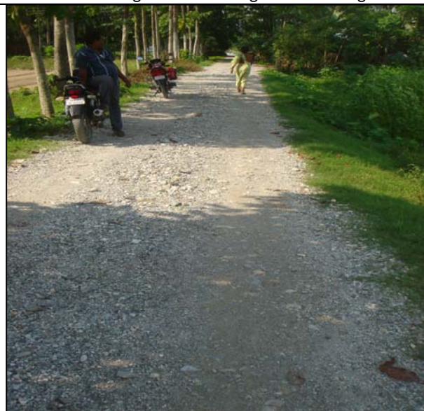
Condition of the road inside the village
