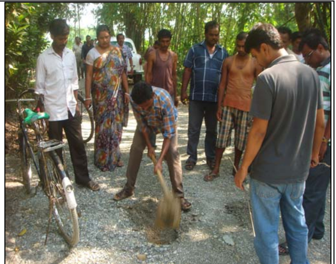
Assistant Engineer assessing the quality of RBM work
